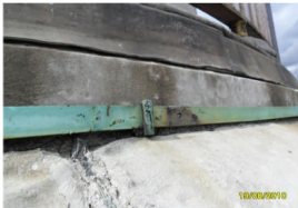
244. lead flashing under asphalt walkway
