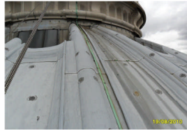
240. Dome Inspection Descent 2 @ SW
